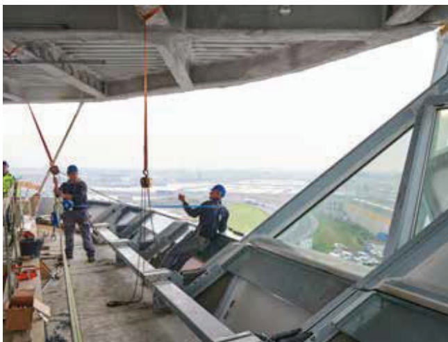
Complex building façades
